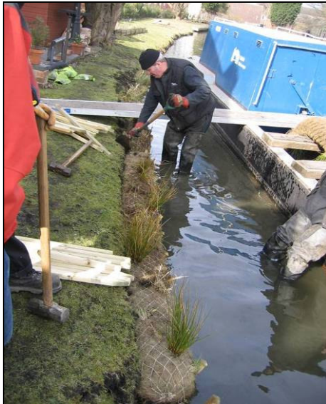
Figure 1.3. Installation of coir rolls
