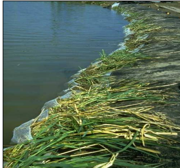
Figure 1.4. Bank reinforced with reed (pocket fabric revetment)
